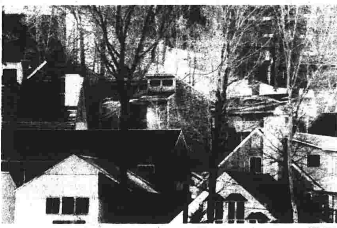
Another condominium takes shape in Sugarbush Village at Warren, Vt., recently. Resort development has come under fire by environmentalists and the Green Mountain State.
